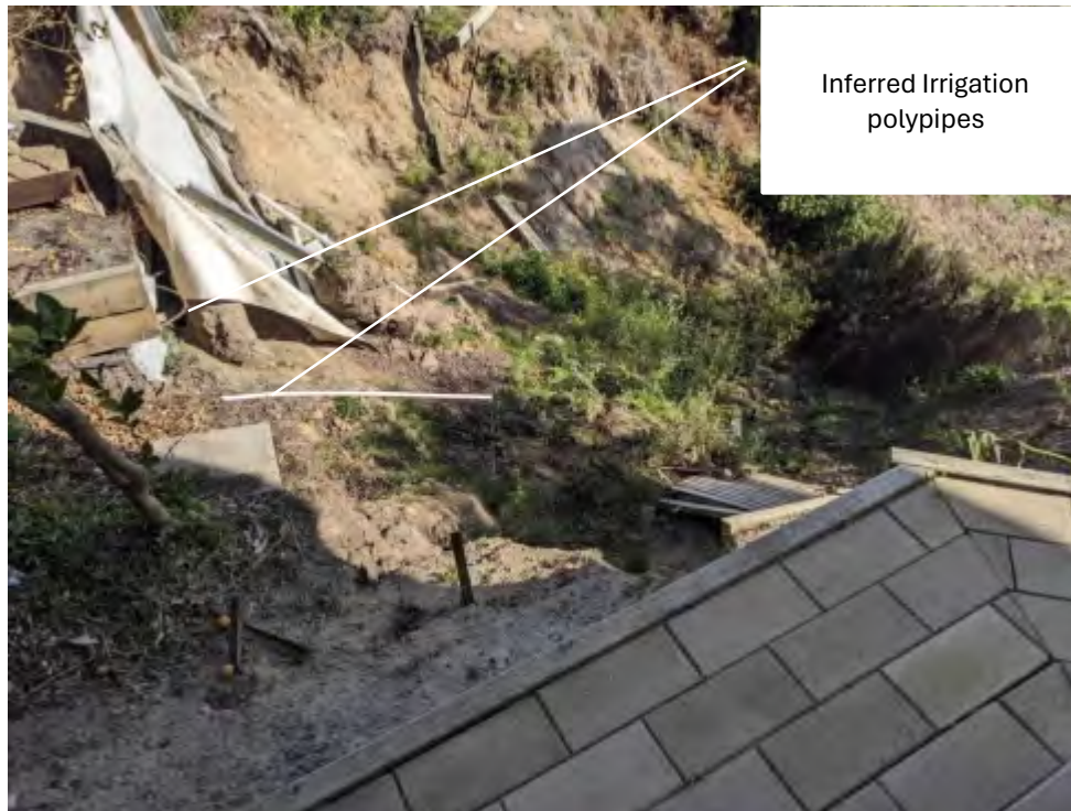
Figure 23: 20/6/25 Looking north west down the failure, showing depth of slope movement.
