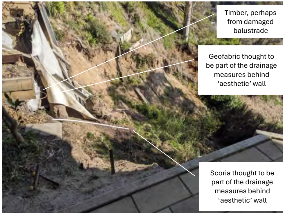
Figure 19: 20/6/25 Looking west showing failed slope material below retaining wall, note the vegetation at the floor of the failed material
