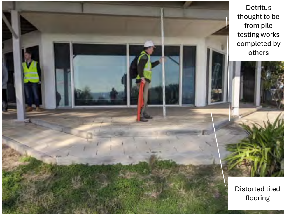
Figure 17: 20/6/25 6 View Point Road, looking south note the disturbed paving, but the house does not show signs of movement.
