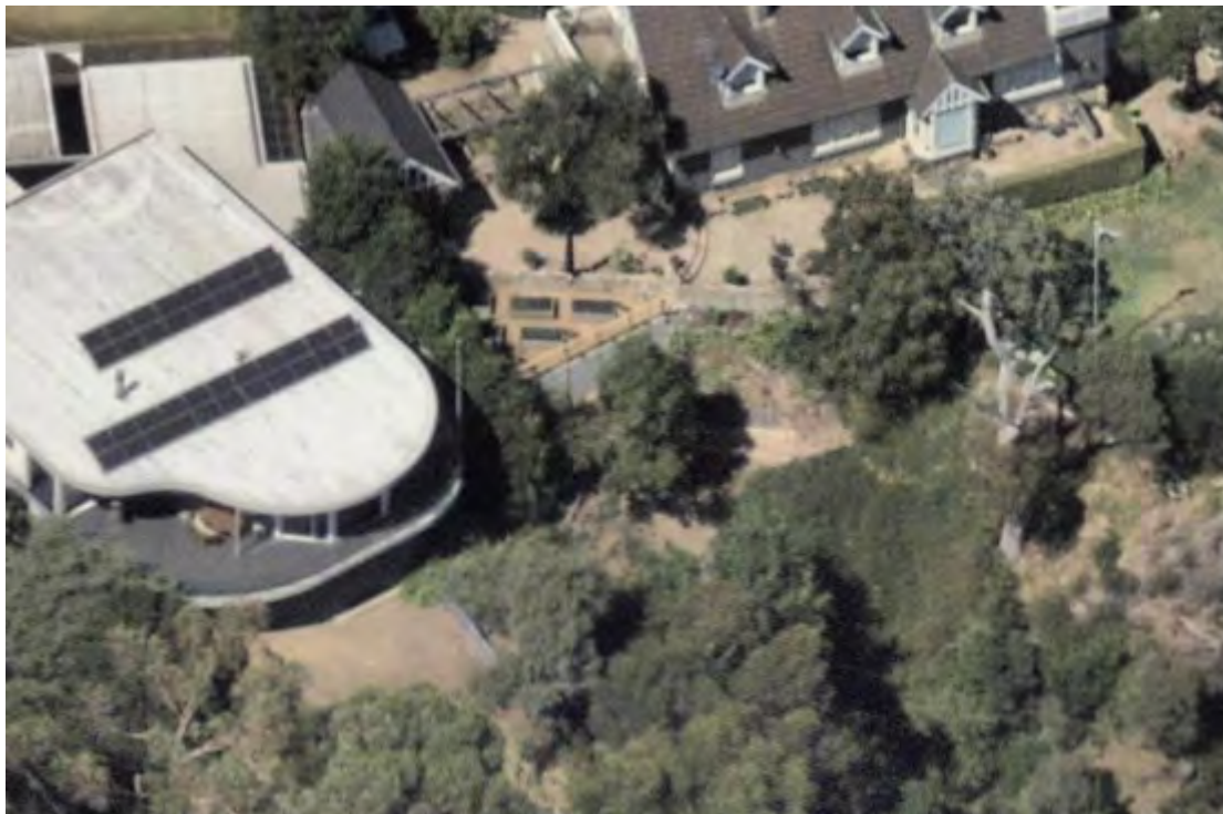
Figure 1: Aerial photo on 15 February 2024 (Nearmap 2024)
