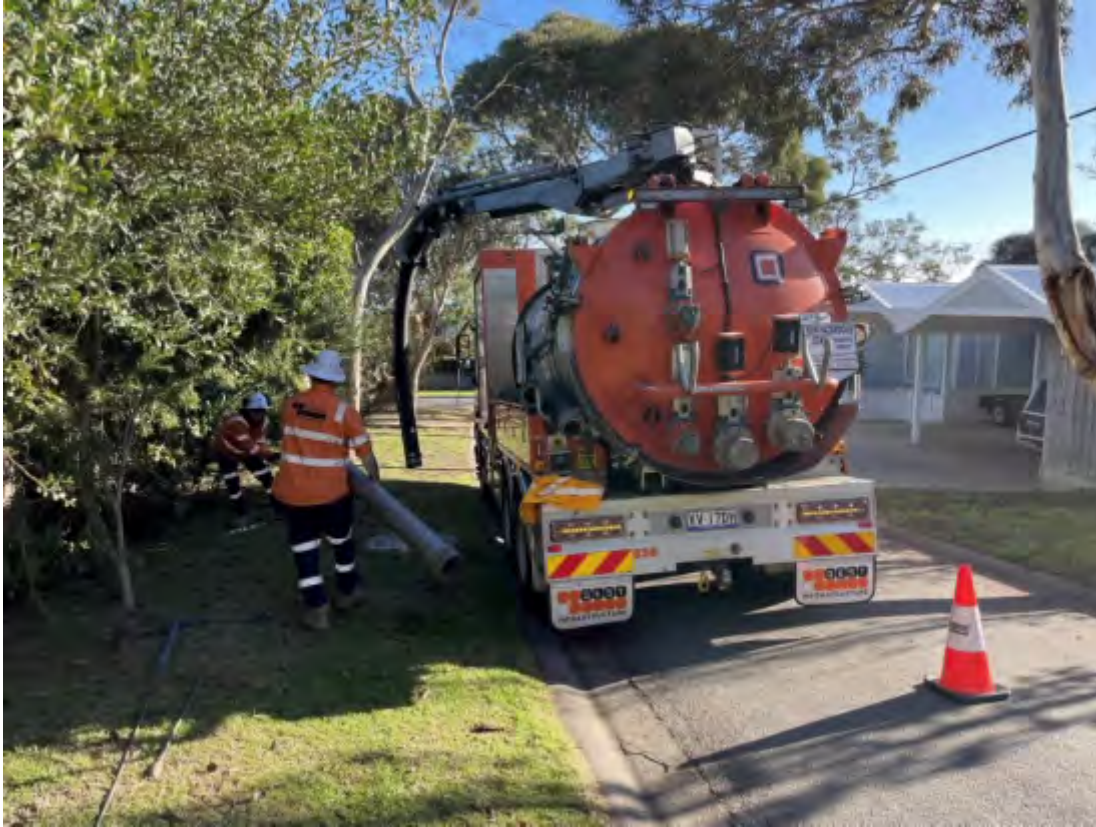
Figure 3: Non-Destructive Digging vacuum truck
