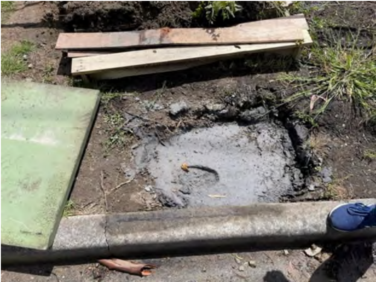
Figure 26: Photograph from email of 22 November 2022, showing detail of sinkhole repair adjacent to a kerb.
