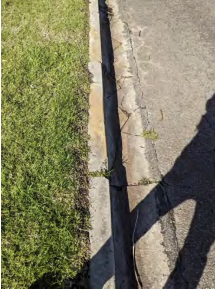
Figure 32: 20/6/25 Looking north from 6 Prospect Hill Road, showing cracking, and staining of kerb suggesting runoff has previously flowed over of kerb.
