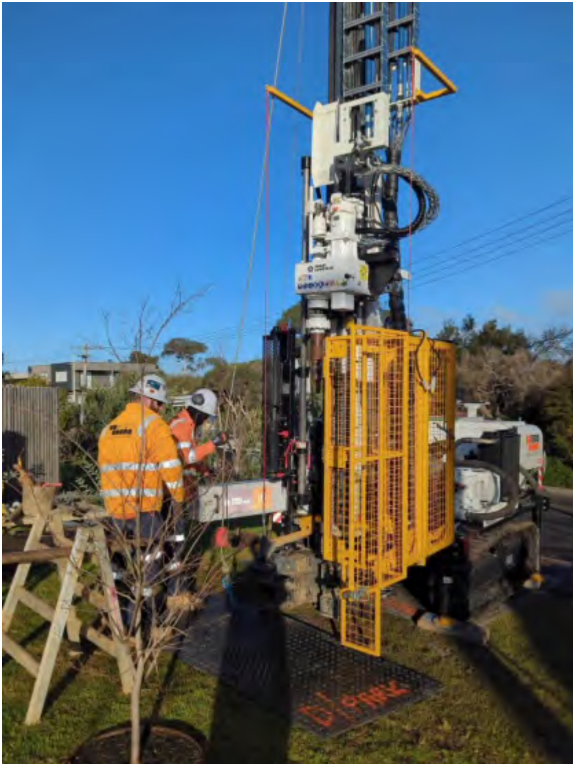
Figure 1: Boart Longyear LX6 drill rig setup
