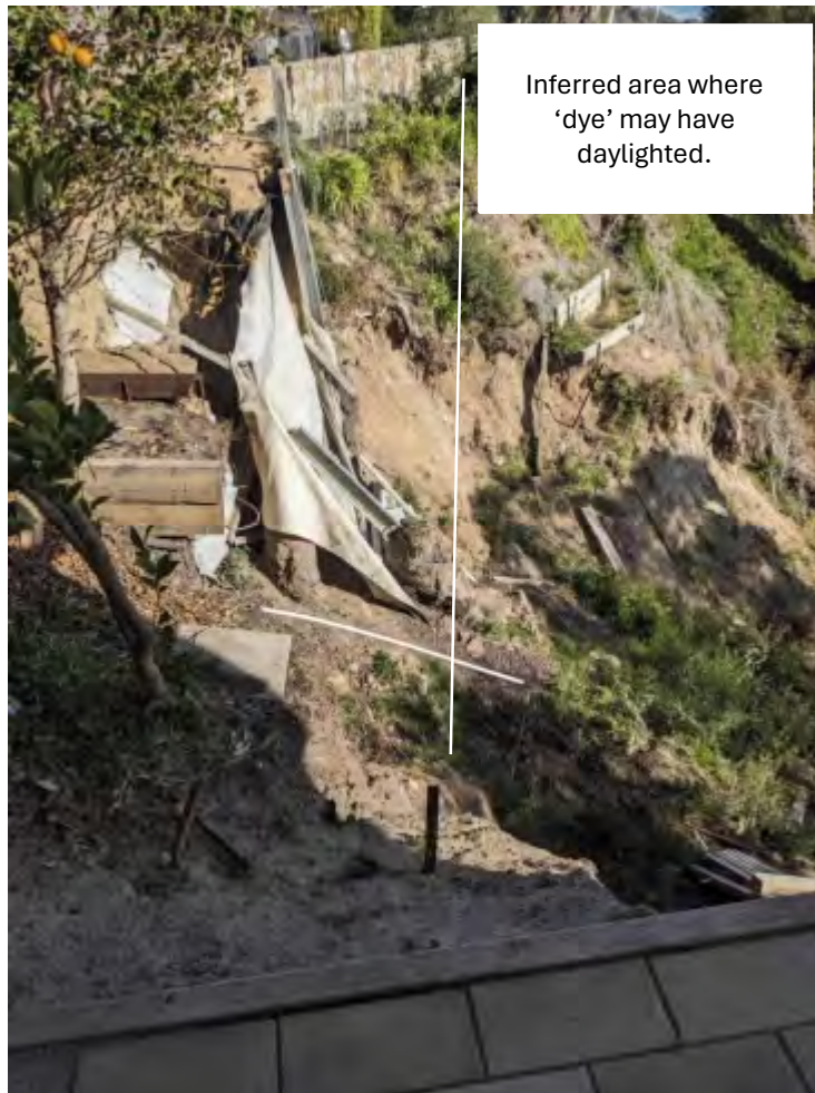
Figure 22: 20/6/25 looking west showing colluvial material exposed , note the geofabric behind the line of the retaining wall.
