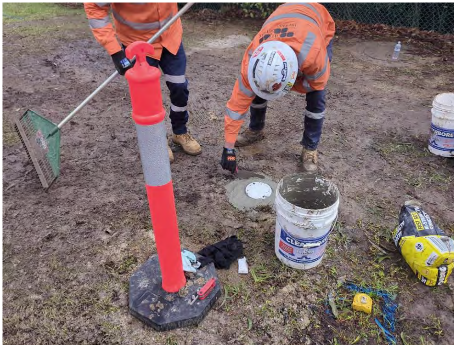
Figure 4: Well installation at BH01
