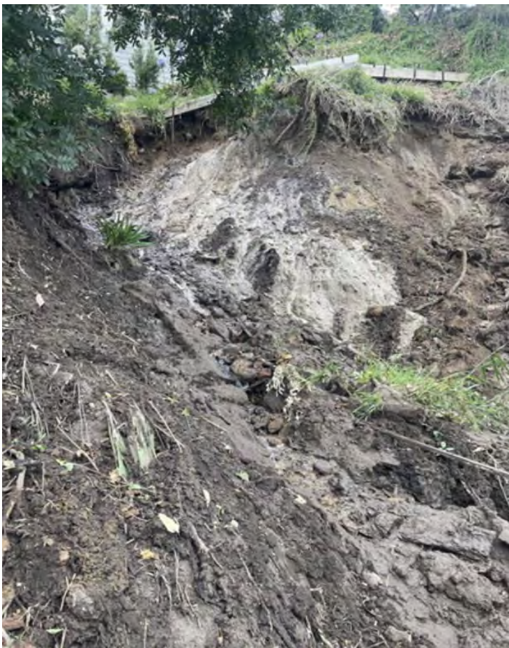
Figure 3: Photo taken by SEW personnel 6 January 2025 showing landslide from midslope of 10-12 View Point Road
