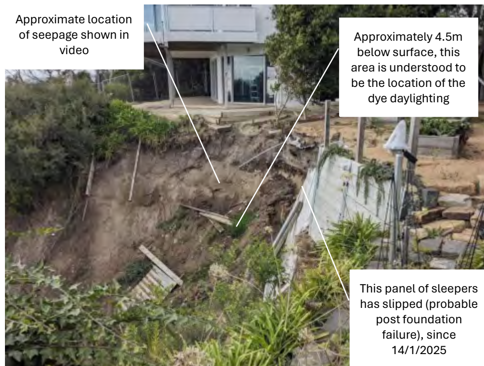
Figure 12: 17/6/25 Photo 09 Looking east showing the location of the seepage videoed by the landowners on 14 January 2025, and location of the dye that was seen daylighting through the backscarp after dye was poured into NDT01/02.
